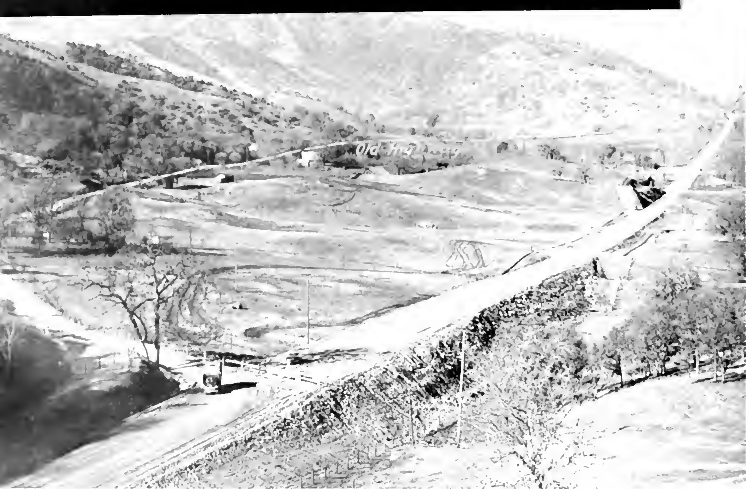
New direct routing of Redwood Highway section north of Hopland in Mendocino County. Dotted line indicates old route through hills.
